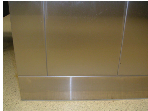
Finished floor detail
